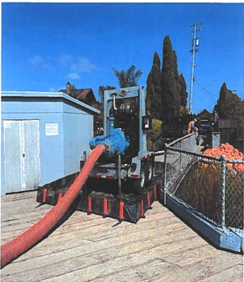
Pump used to dewater the North lock
