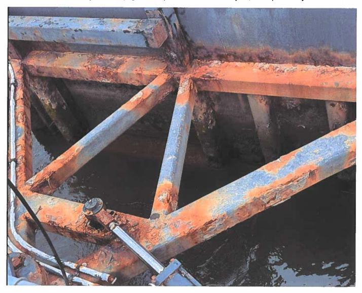
The framework for the South lagoon-side lock is so heavily rusted that holes are appearing in these large beams. There is concern that the actuator force required to open and close these locks will tear a rusted section out of these beams, leaving the lock inoperable.
