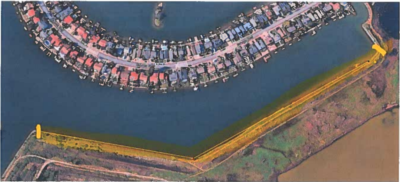
Image 1. Work Area Highlighted in Yellow – 2,700 LF on the Levee Slope
